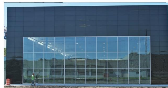
PV Curtain Wall by BISEM at Guardian Industries Science and Technology Center in Detroit, Michigan
